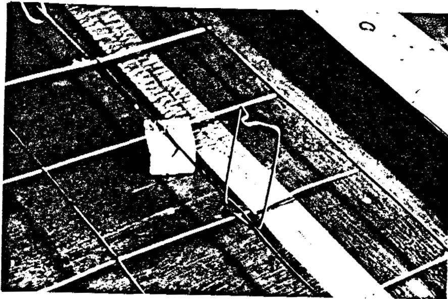
Fig. 4 Mounting of Type A-3 Metal Tie to Wire Mesh for Wall P2
