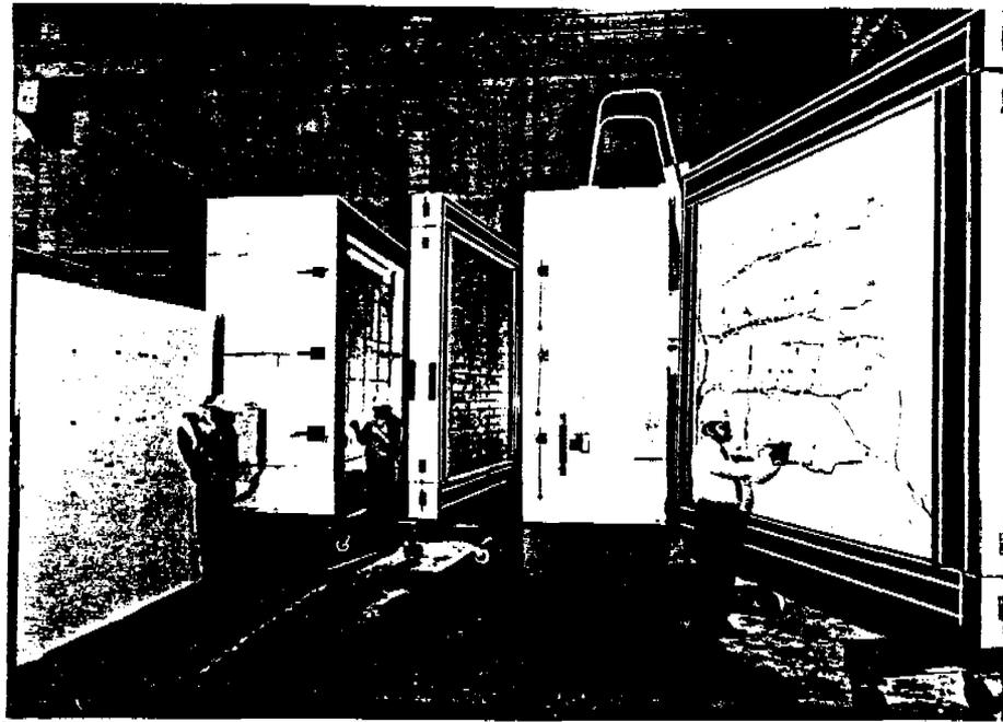
Fig. 6 Calibrated Hot Box Test Facility
