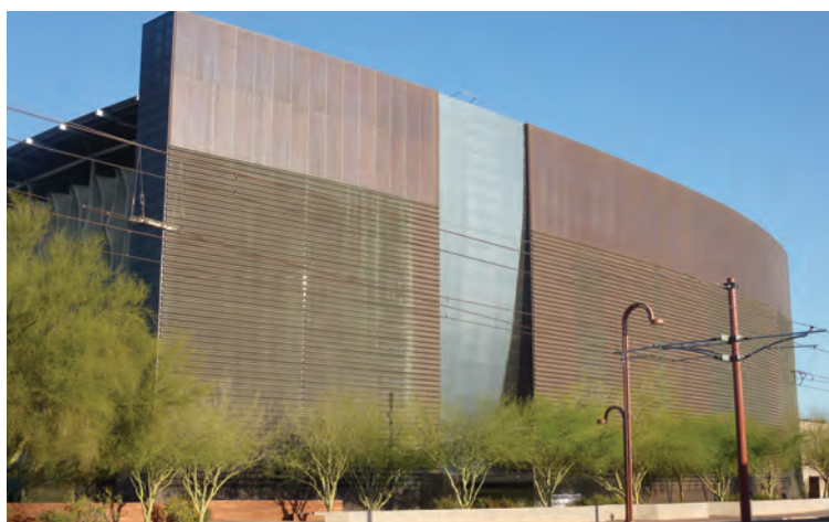
Photo 1 (left) West wall protection in Climate Zone 2 (photo: Will Bruder + Partners).
