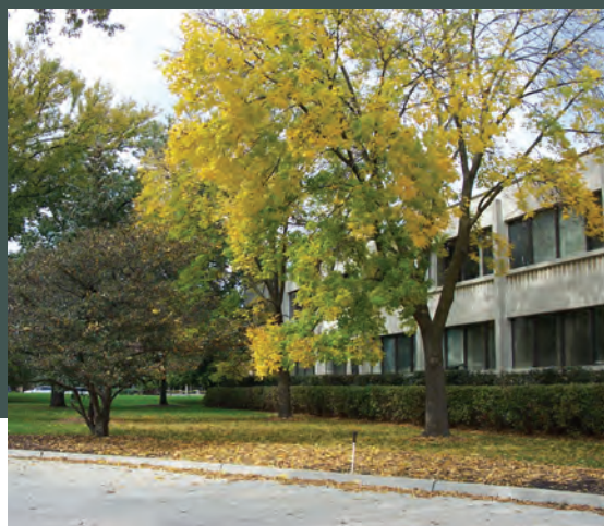
Photo 2 (below) Shade on the west wall in Climate Zone 5 (photo: CTLGroup).
