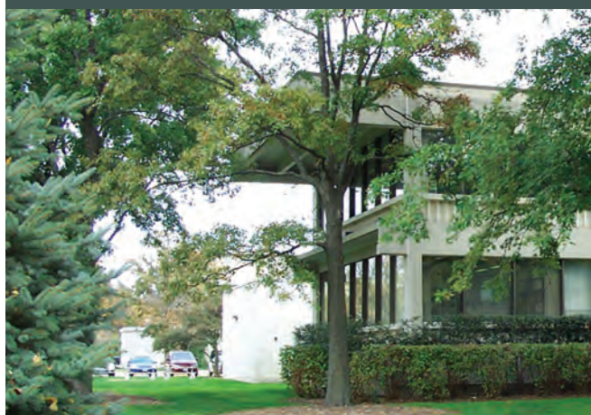
Photo 1 Overhang on west face of building in Climate Zone 5 (photo courtesy of CTLGroup).
