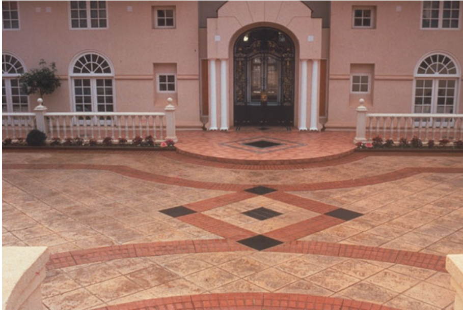
Fig. 6 Decorative flatwork combining plain concrete, textures, exposed-aggregate, pattern stamping, divider strips, and borders (Photo courtesy of the Portland Cement Association, www.cement.org , Nos. 9046)
