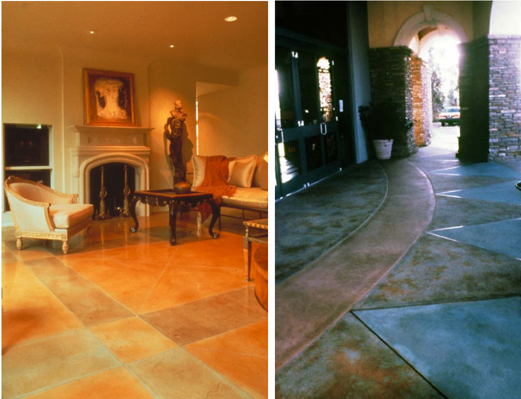
Figure 8. Stained concrete on interior floor. (Photos courtesy of the Portland Cement Association, www.cement.org , Nos. 5074 and 15195)
