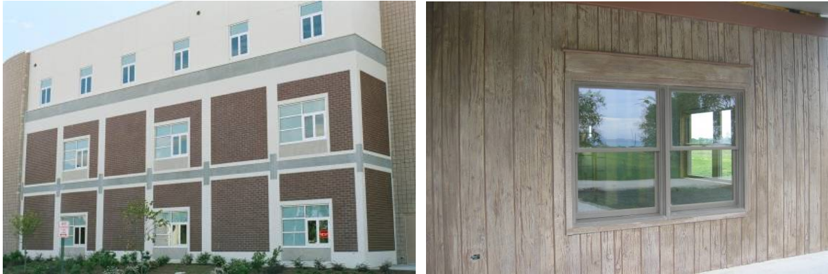
Figure 4. Exterior finish as part of exterior precast wall (a) Simulated brick (Photo courtesy of Thermomass® Building Insulation System www.thermomass.com ) (b) Simulated wood (Photo courtesy of Dukane Precast, Inc www.dukaneprecast.com )
