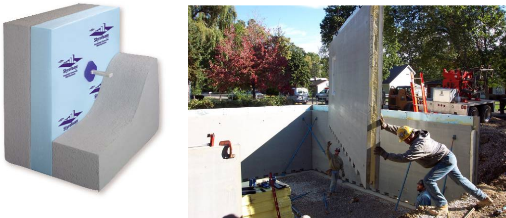
Figure 3. Precast sandwich panel wall with a layer of insulation between two layers of concrete (a) with low conducting fiber composite connectors (Photo courtesy of Thermomass® Building Insulation System www.thermomass.com ) (b) being set into place (Photo courtesy of Dukane Precast, Inc www.dukaneprecast.com ).
