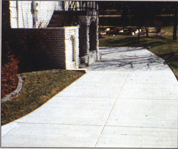
This sidewalk of white portland cement illustrates the use of a light-coloured, high-albedo material for at least 30 per cent of the site's impervious surfaces.
