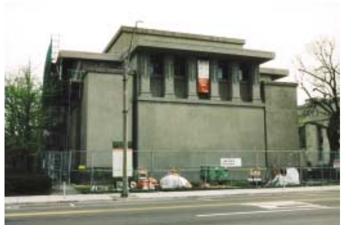
Fig. 3: Renovating an existing building and leaving the concrete shell in place
