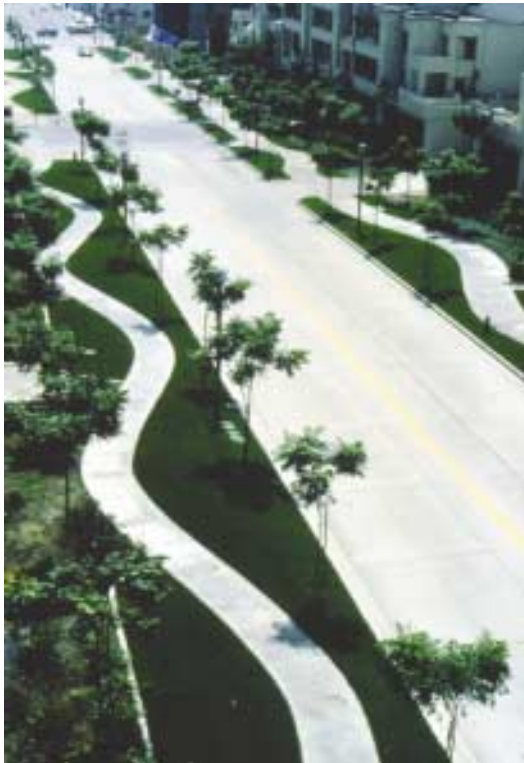
Fig. 1: Concrete pavement and trees used to mitigate the urban heat island effect (Photo courtesy of the Portland Cement Association)
