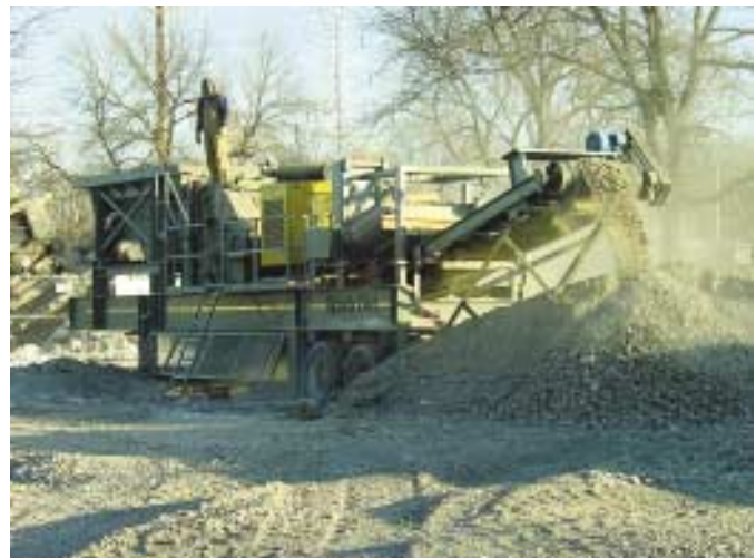
Fig. 4: Crushing concrete for reuse as fill or road base
