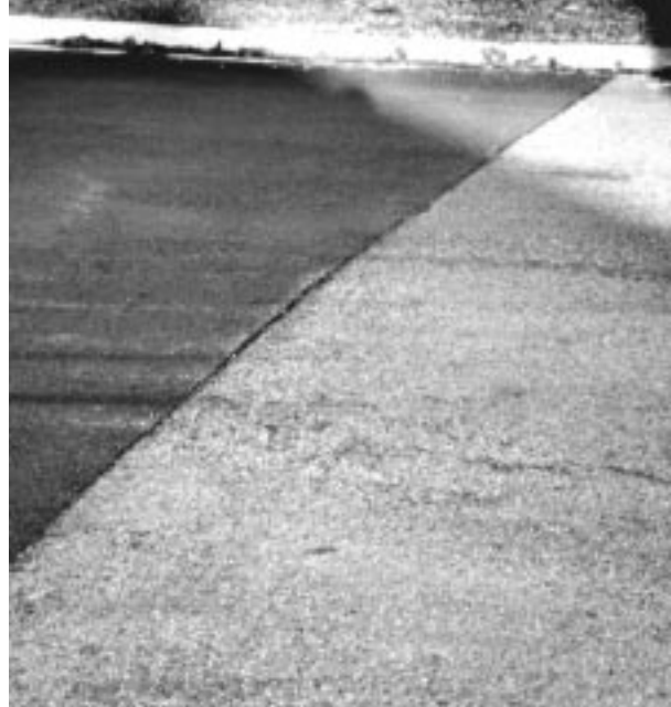
Figure 3. New ACC pavement on left, old ACC pavement on right.
