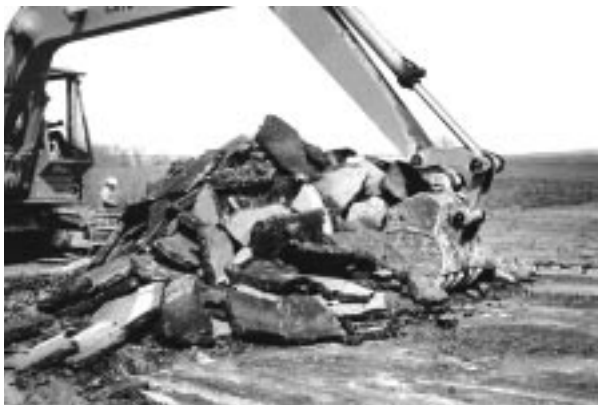
Figure 13. Removal of ACC pavement for recycling. (S-38441)
