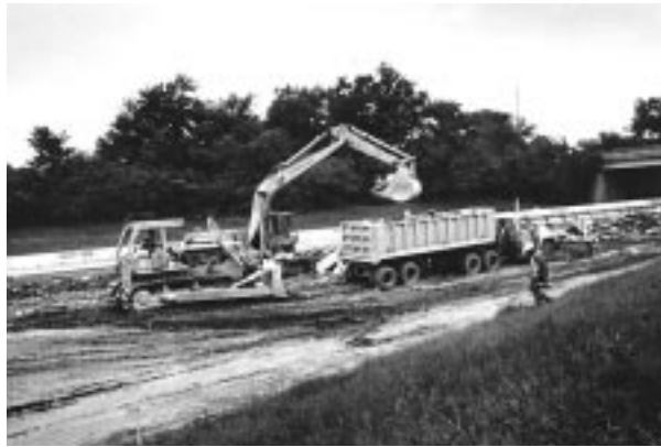
Figure 10. Removal of PCC for recycling. (S-42534)
