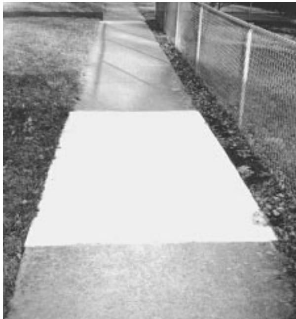
Figure 2. New PCC section in weathered PCC sidewalk.
