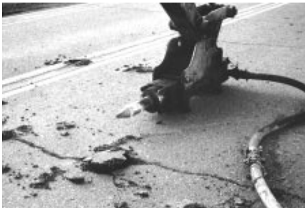
Figure 12. Loosening of ACC pavement before removal. (S-39363)
