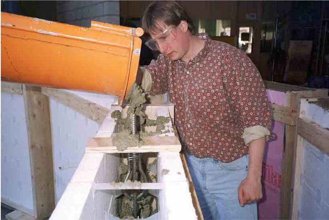
**Figure 10. Placement of concrete into ICF.**
