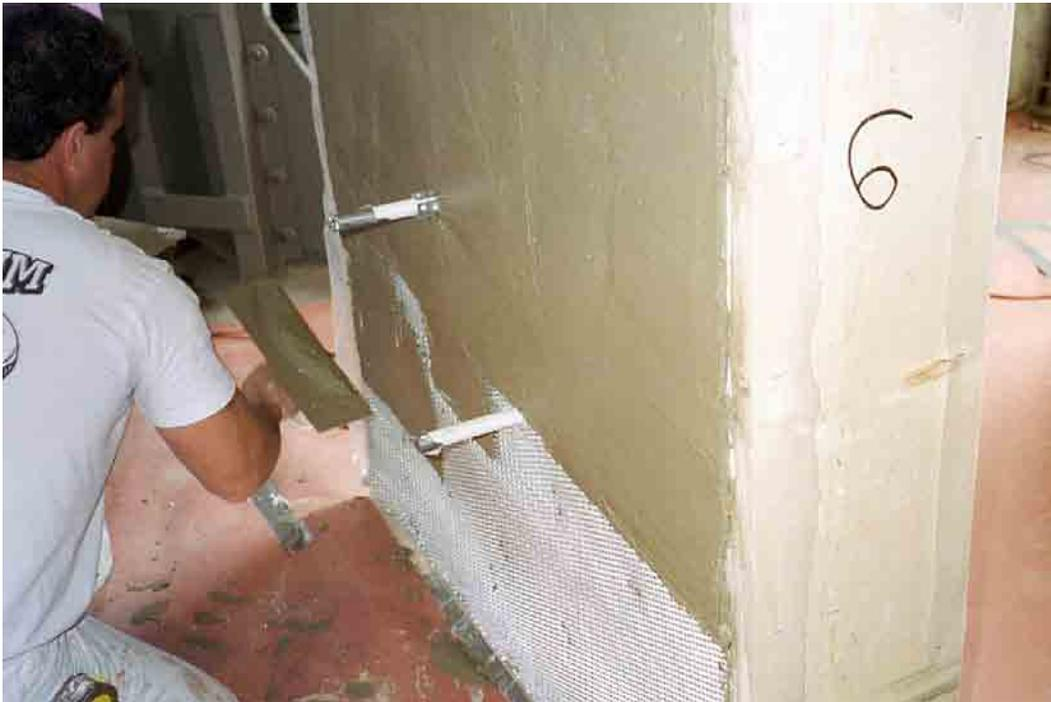
**Figure 22. Application of portland cement stucco base-coat.**
