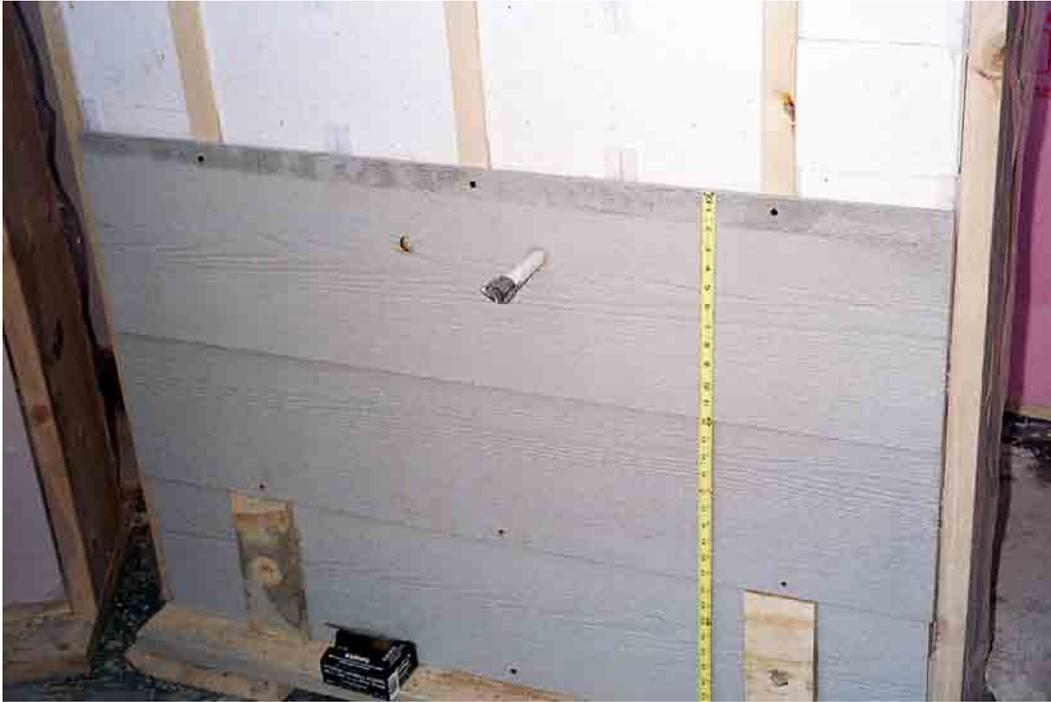
Figure 16. Installation of hardboard lap siding on wood furring.
