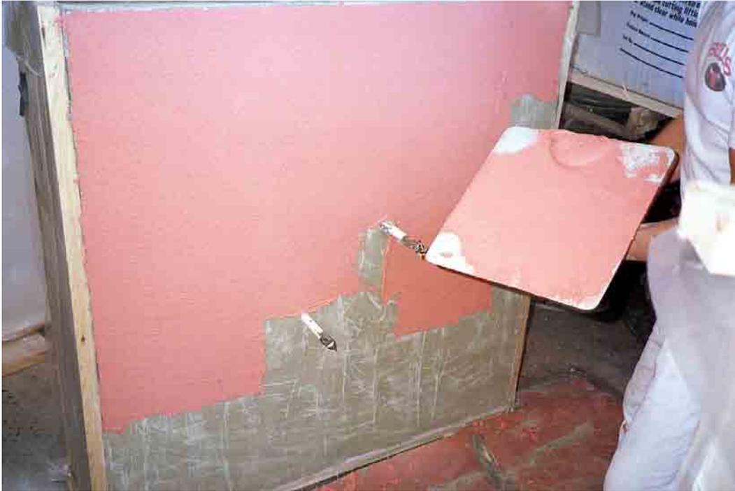
**Figure 20. Application of the EIFS top coat.**
