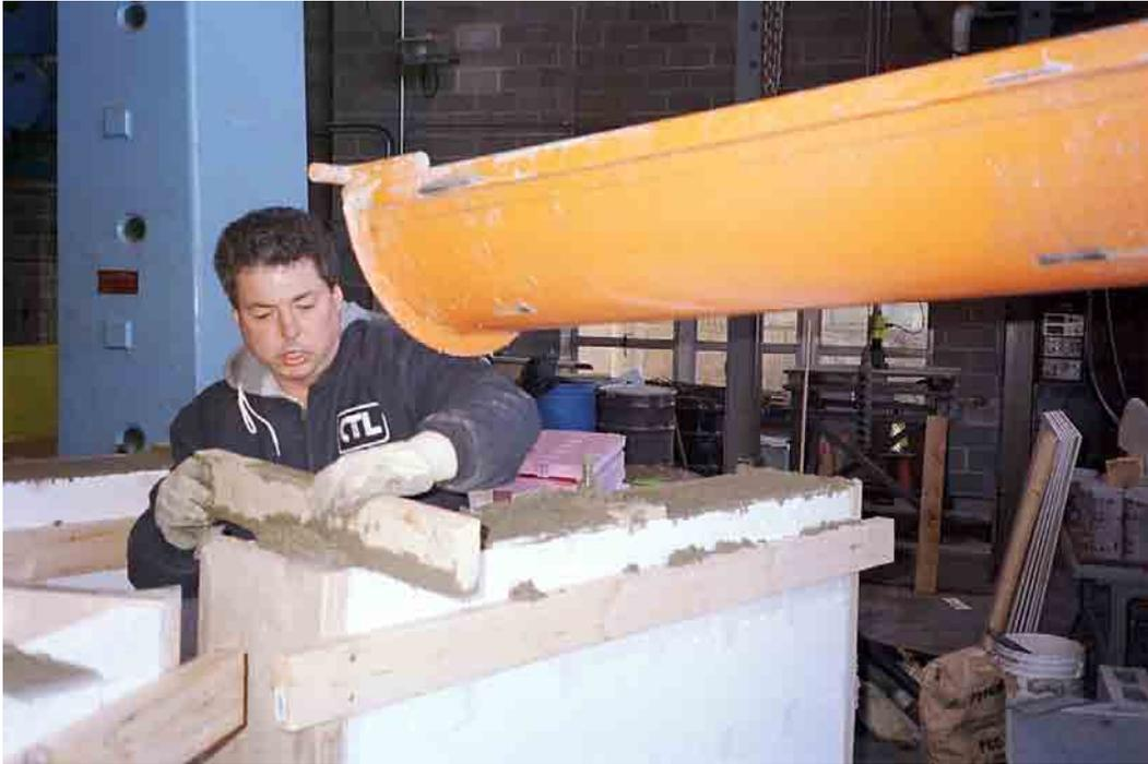
Figure 12. Strike-off of concrete.
