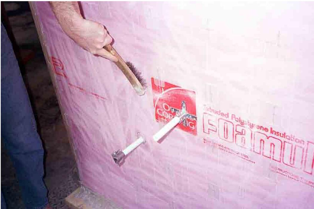
Figure 17. Roughening of XPS insulation prior to application of the EIFS base coat on Wall No. 1 (NOT A RECOMMENDED PRACTICE).
