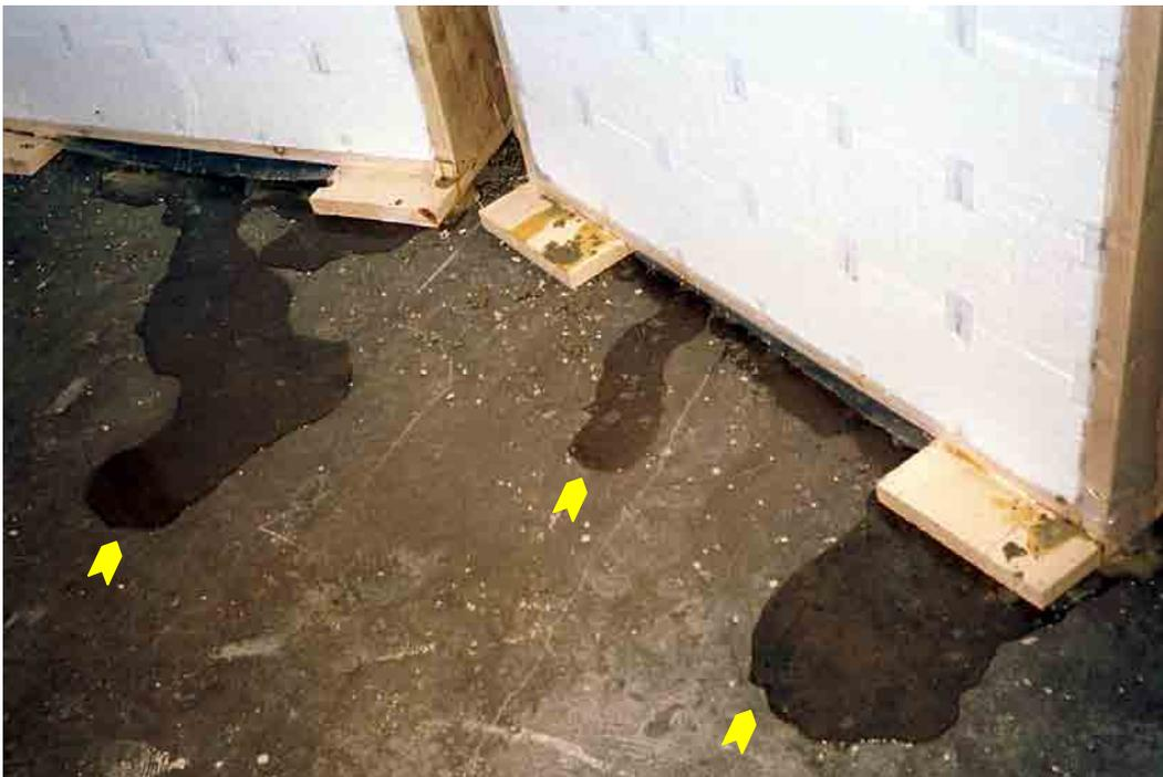
Figure 13. Mix water leaking from ICF walls immediately after casting.
