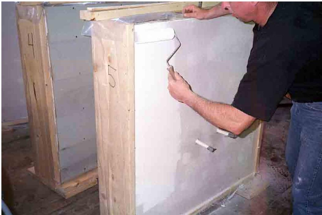
**Figure 15. Application of latex primer on finished drywall.**
