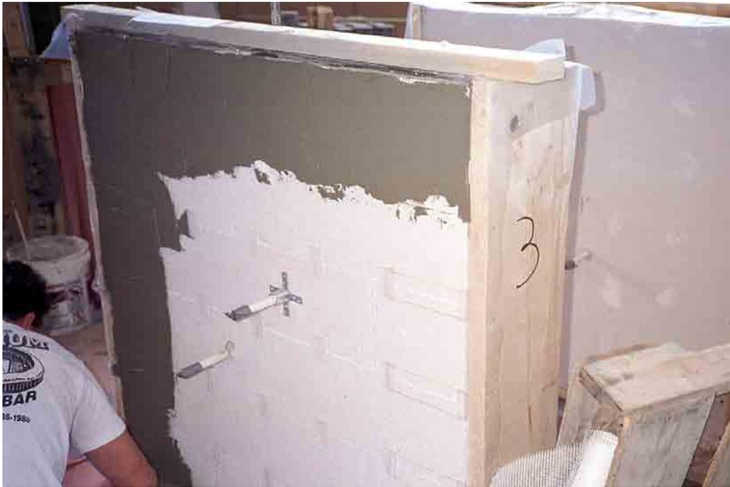
**Figure 18. Application of the EIFS base coat on EPS insulation of Wall No. 3.**
