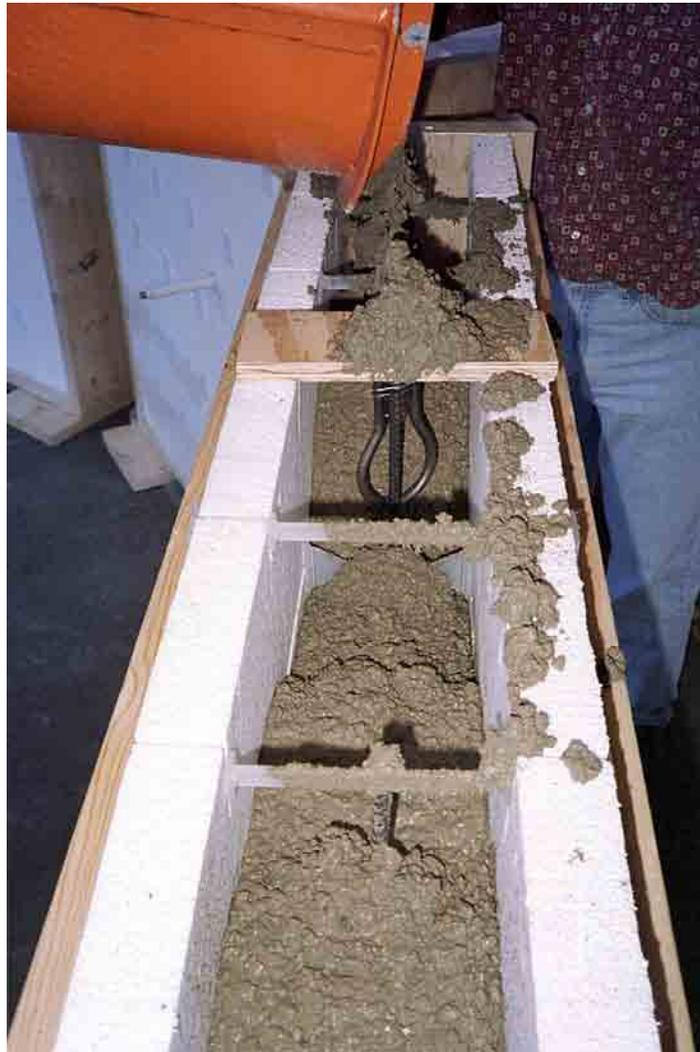
**Figure 11. Close-up of placement of concrete into ICF.**
