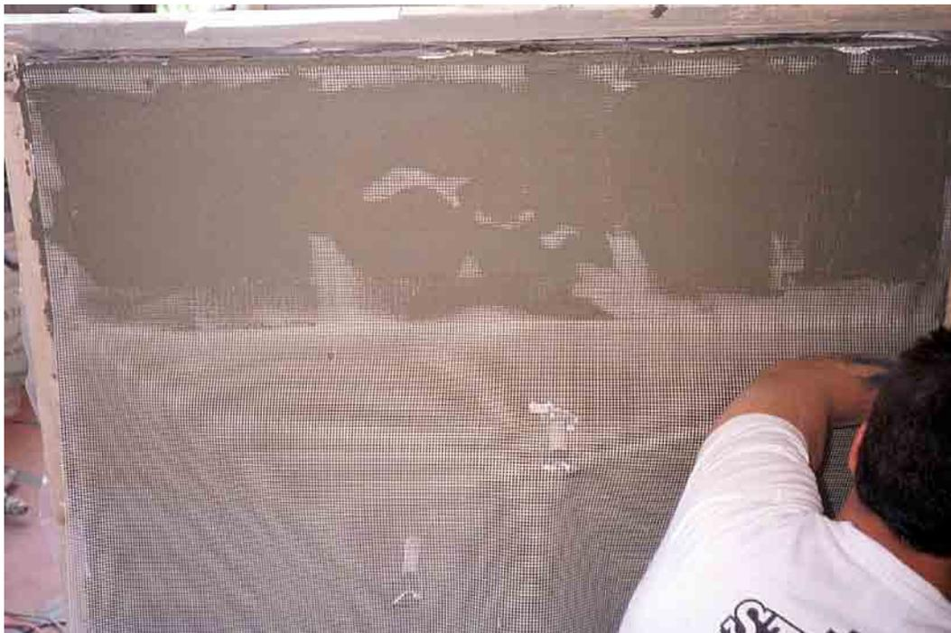
**Figure 19. Application of fiberglass mesh into the EIFS scratch coat.**
