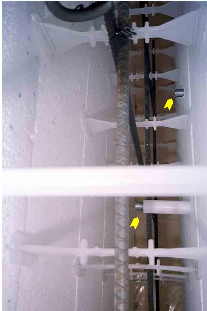
**Figure 9. Temporary plugs installed in the relative humidity measurement ports at the concrete–insulation interface and center of concrete in Wall No. 1.**
