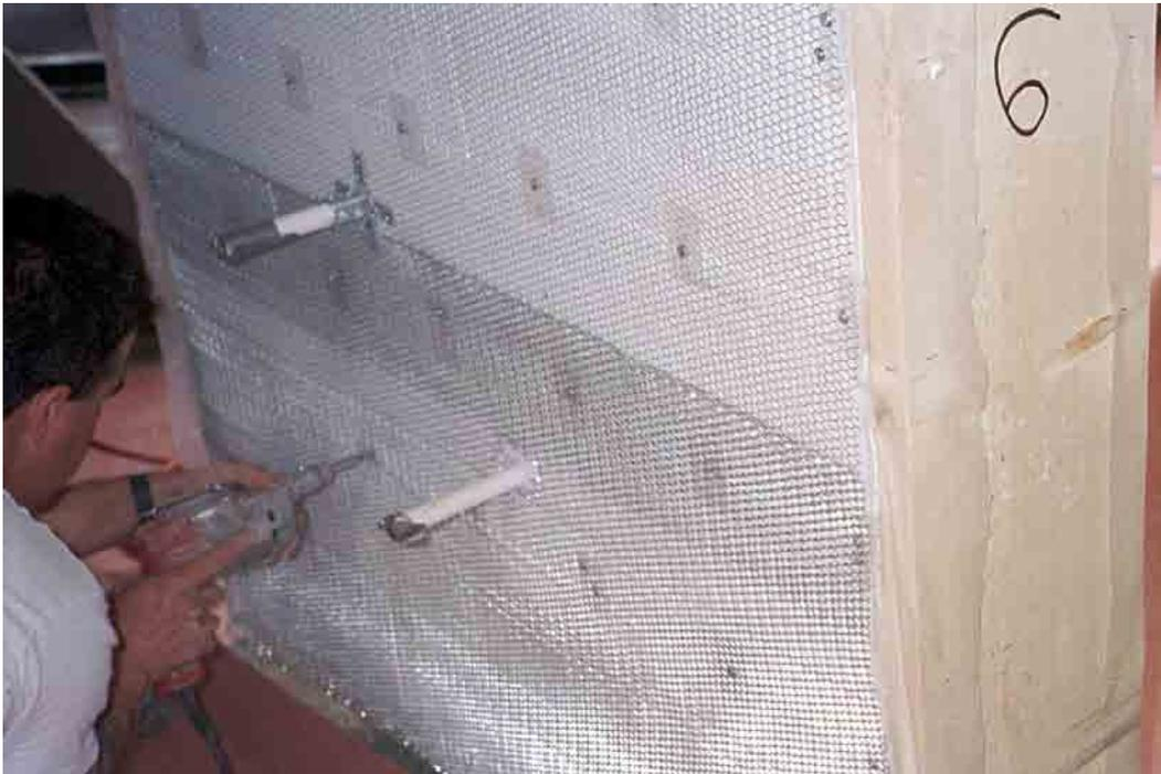
**Figure 21. Application of metal lathe prior to portland cement stucco.**
