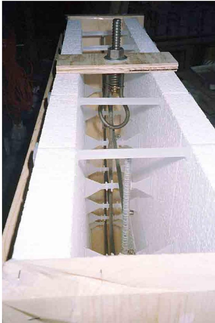
**Figure 4. ICF wall section with reinforcing steel and lifting lug installed.**
