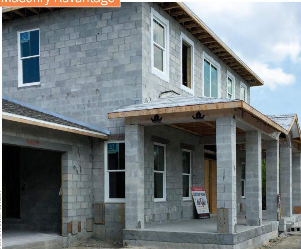
CMU structural walls provide thermal mass to reduce the amount of insulation needed in comparison to wood-frame walls.
