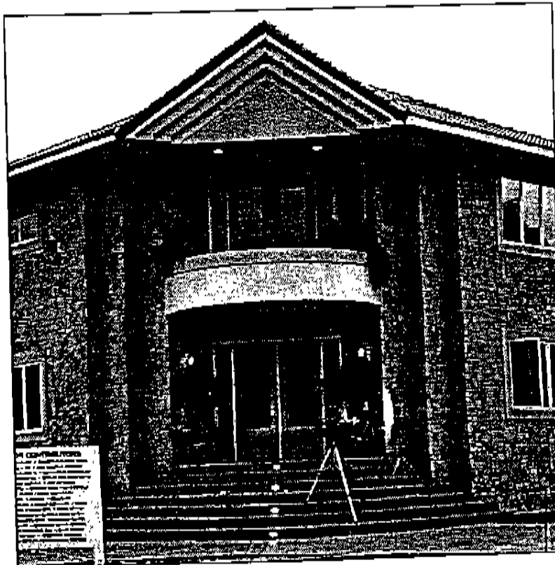
Fig. 5 Home Constructed of ICF's After Exterior Finish is Applied (PCA No. 67366)
