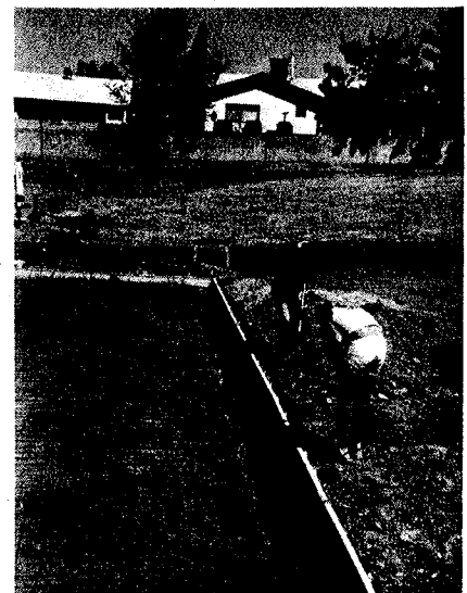
System 150: insulated slab edge with exterior protective coating
