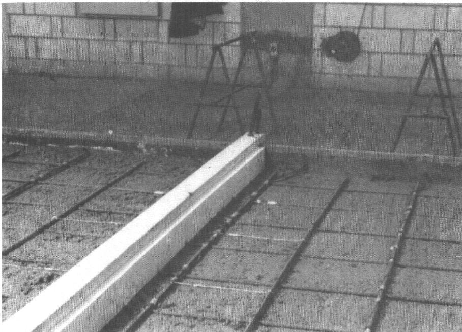
Fig. 5 Reinforcement Placed over First Layer of Concrete for Wall S
