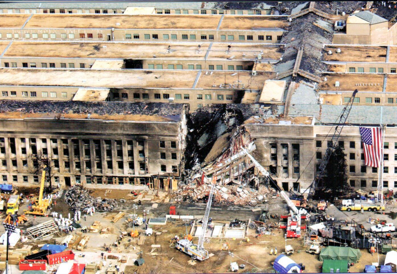
Figure 8 – Damage from impact and blast due to terrorism at Pentagon on September 11, 2001. (Image 60569, www.pixabay.com )
