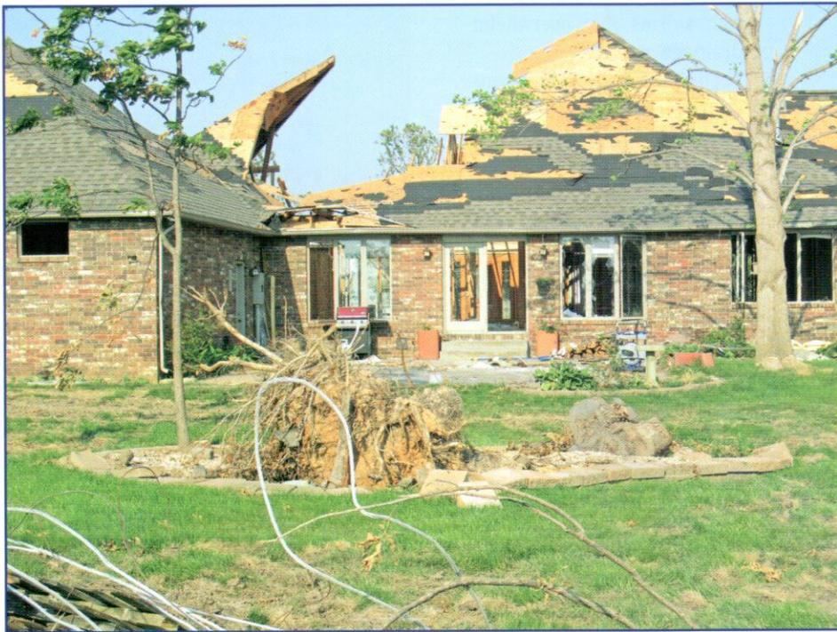
Figure 5 – Wind damage to house caused by tornado in Joplin, MO. (Image 642586, www.pixabay.com )
